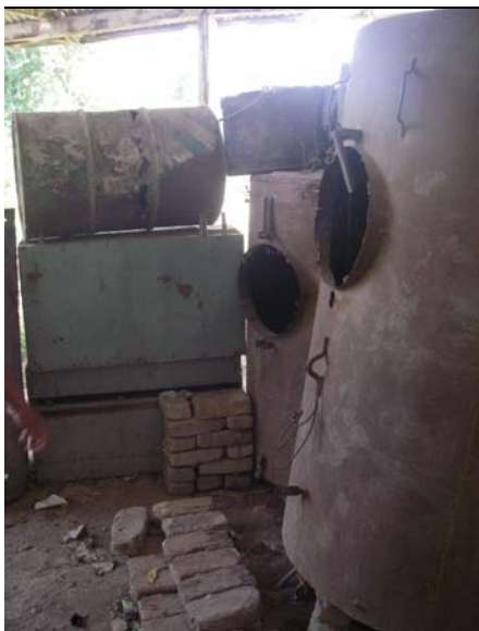
Figure 4.12 Shower partly constructed from empty drums / tanks used to store pesticides
