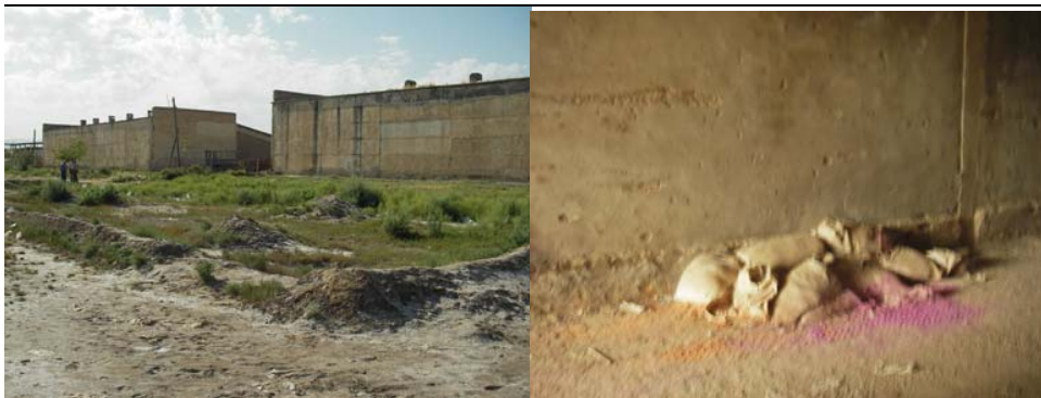
Figure 4.2 Old basin and obsolete pesticides in Paiskambe 2
