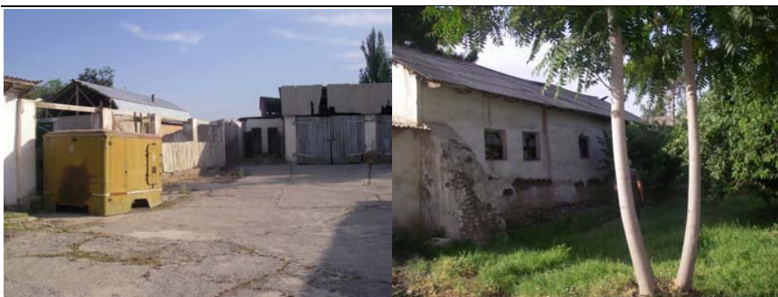
Figure 4.8 Overview shed 3 and 4 at the back left and overview backside storage room 1 and 2
